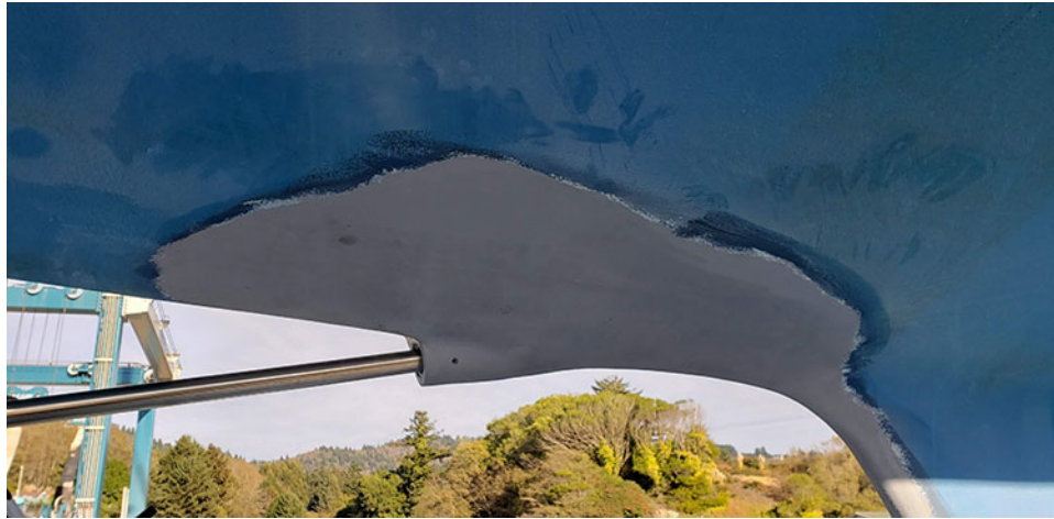
First barrier coat applied.
